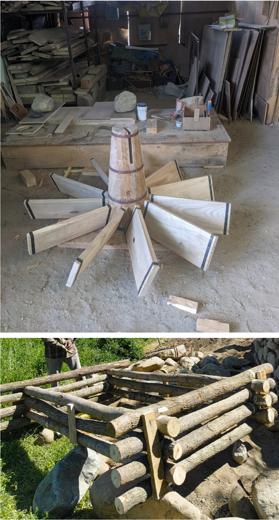
Turbine and door frame ready to be assembled at the site. Images: Field Studios
