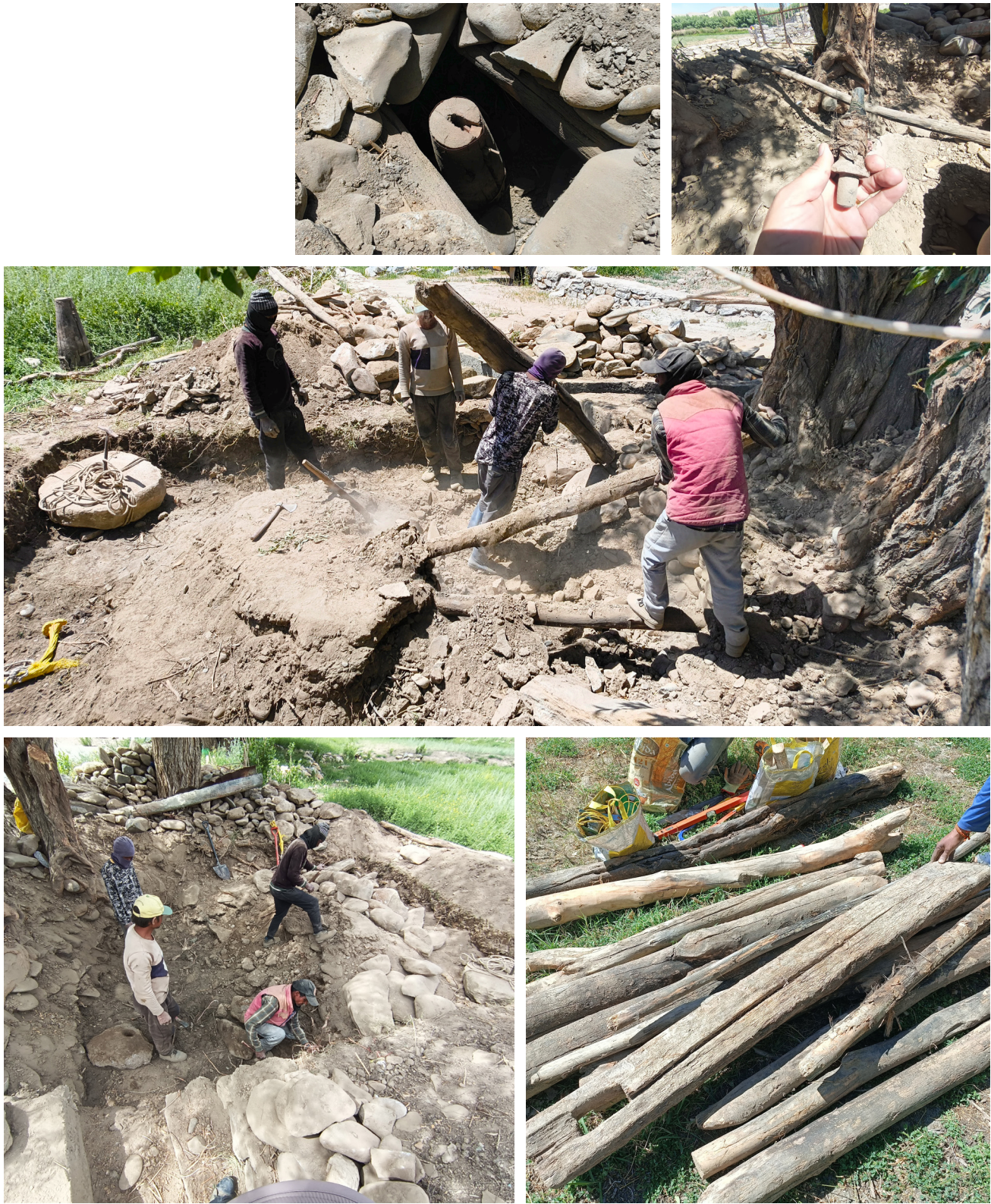
First row (left and right): Decayed turbine (skuru) removed for study and replication; spindle (phang) cleaned for reuse. Second row: Poplar trunks (dungma) extracted, most of them reused within the new structure Third row: Foundation base excavated deeper for improved stability as well as soling. All wooden members extracted. Images: Field Studios
