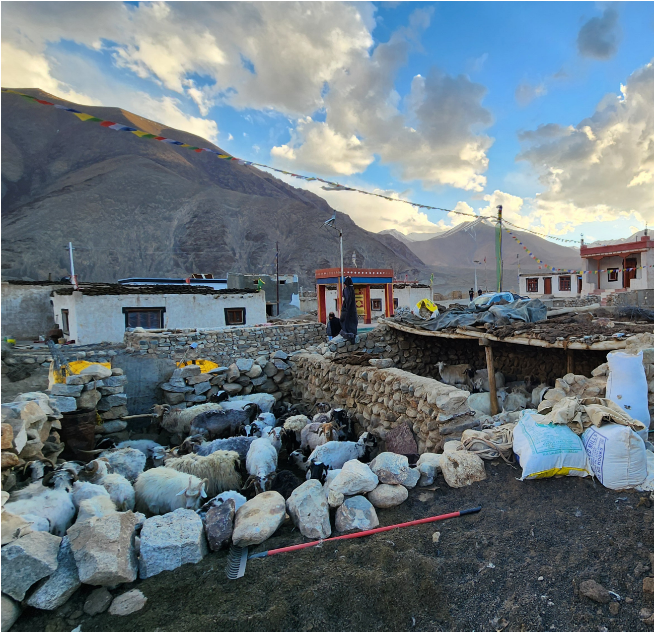
(Below) Winter corrals made with stone and mud, with open tops in Chibra village. The area marked by the red stick is where pastoralists used to sleep to guard their livestock from predators. These corrals are now upgraded under the project, removing the need for night guarding in winter. Image: Saloni Bhatia
