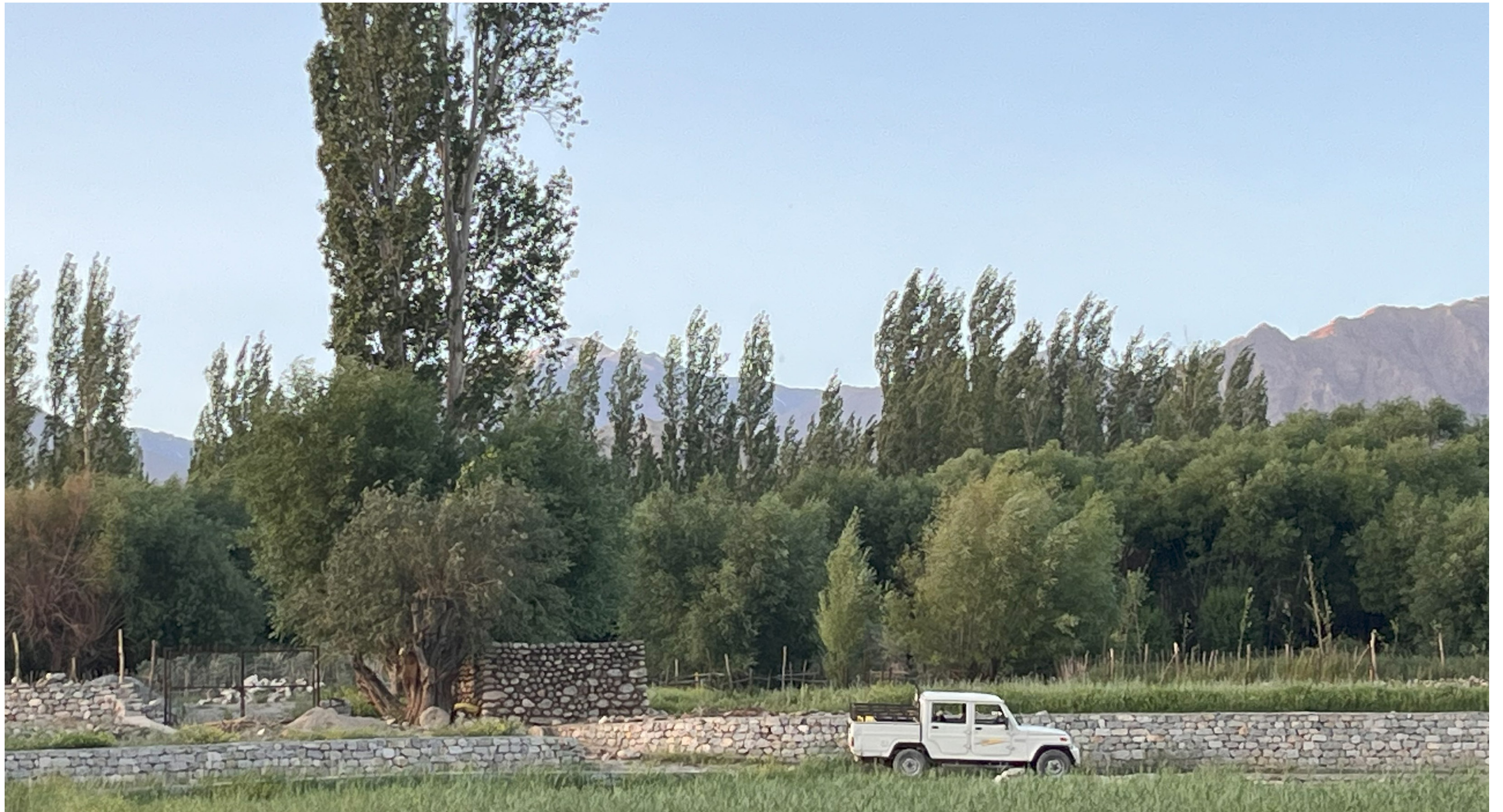
The completely restored Sintik rantak, with its organic river-stone masonry, sits discreetly within the village landscape. Photo: Field Studios
