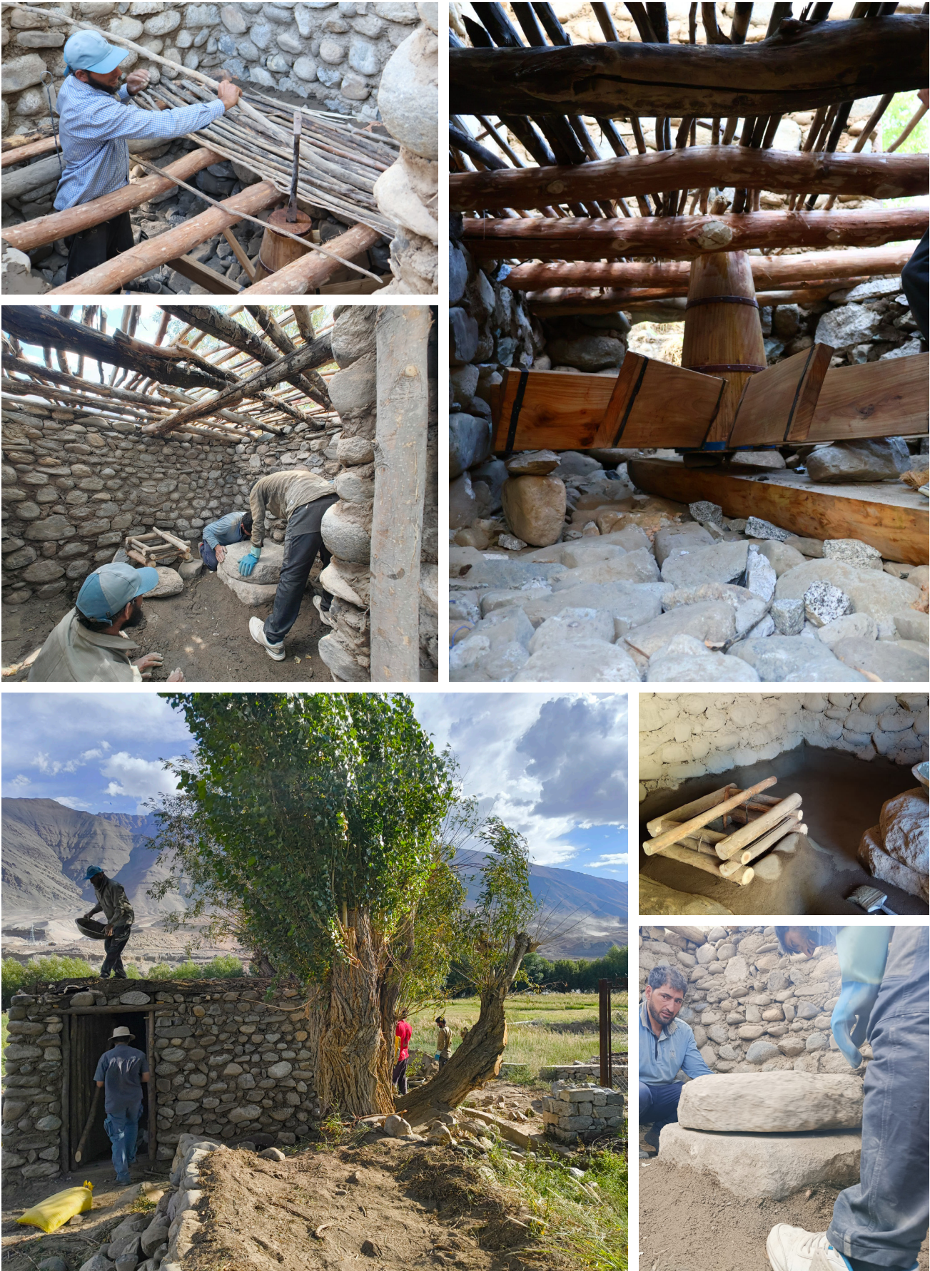
Internal parts of rantak being re-installed at site along with the finalisation of structural work. Images: Field Studios
