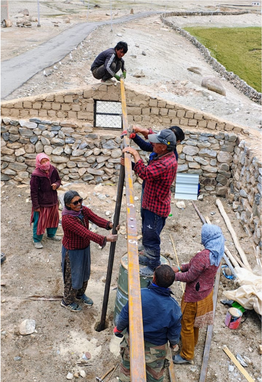
The work started in the last week of May 2025 by contractor Konchok Sangrob and executed by Rinchen Namgail. Photos: Ragav Verma and Rinchen Namgail
