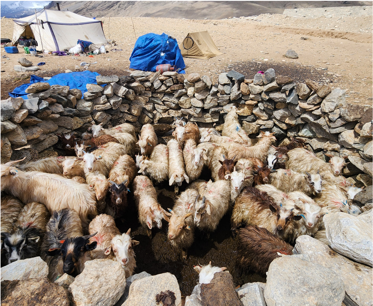
(Image on the next page) Redesigned corral with stone and mud base, and mesh roof. These corrals are used both in summer and winter months. Photo: Rinchen Namgail
