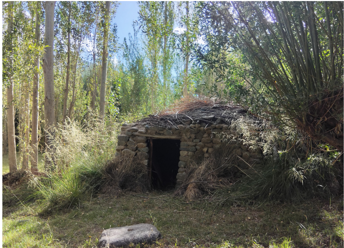
The rantak concealed in dense vegetation, and its roof loaded with dry leaves and twigs. Images: Field Studios
