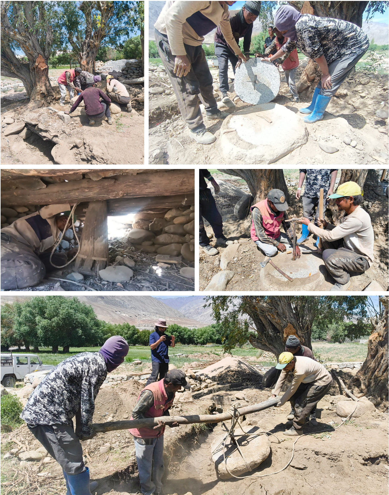
First row: The walls and foundation dismantled; retrieved stones neatly stacked for reuse. Upper stone (kongdo) removed and set aside. Pictures in the second and third row show the process of dismantling the lower stone (yokdo) from the site. Images: Field Studios
