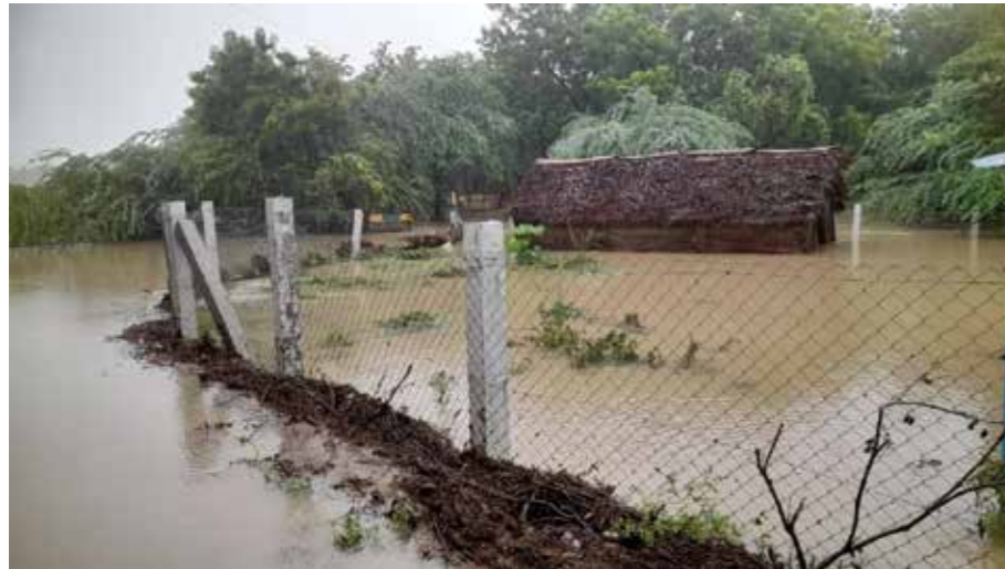
Flooded waste segregation site observed on December 13, 2024, in Thirupudaimaruthur.
