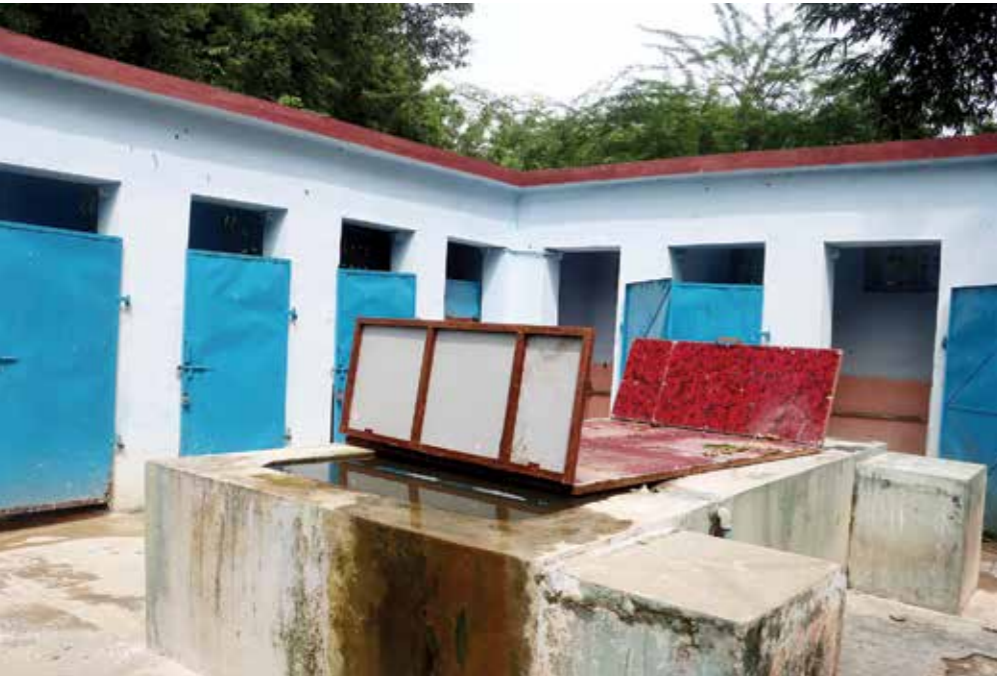
Community toilet complex located near the TBCR premises in Thirupudaimaruthur hamlet.
