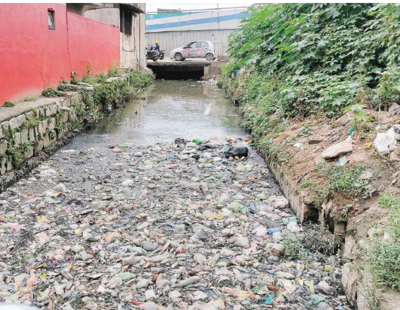
Plate 1-1: Stormwater drain choked with solid waste
