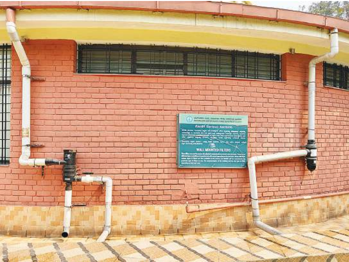
The wall mounted filters for rain water harvesting
