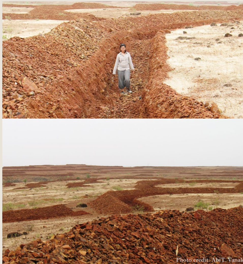
Figure 6: Deep continuous trenching in the grasslands of Manmad in Nashik district. Given the low rainfall and flat topography of this landscape, such massive soil disturbance can do far greater damage to SOC, hydrological cycles and soil health than any marginal benefits derived from greater water retention in the landscape
