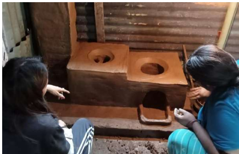
ICS Unit being installed
